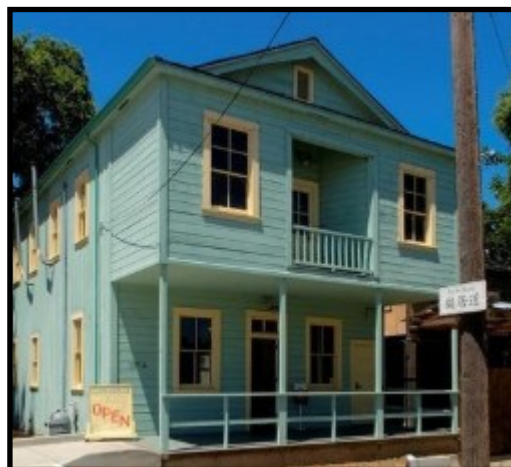
Locke Boarding House
